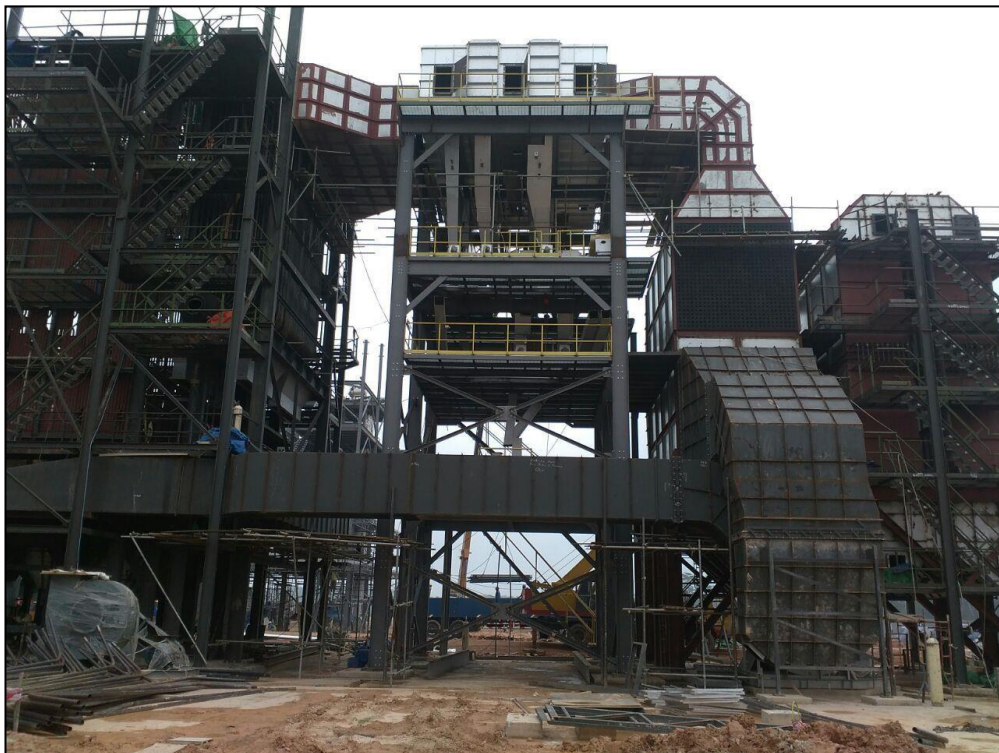
Figure 3: A Modern VORSEP TAS100 filter system on a Palm Oil Boiler
